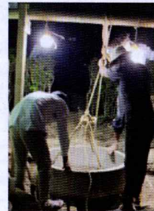
Open Doors partners helped to repair the well
